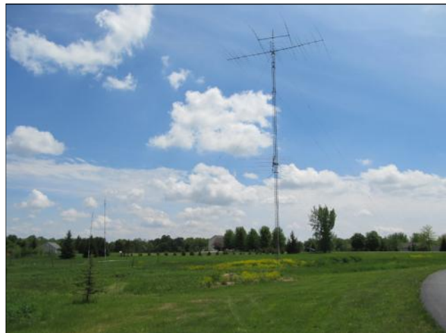
My latest station improvement: 100-ft. Rohn 45G with Yagis (see text, below).
