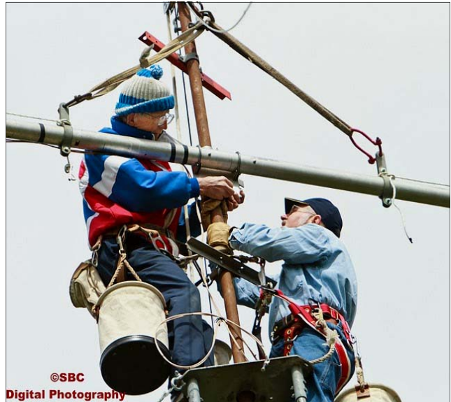
The A-Team in action at the top of the tower.
