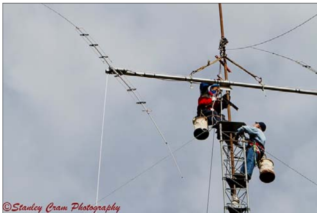
Paul and Glenn position and place the 40m Yagi.
